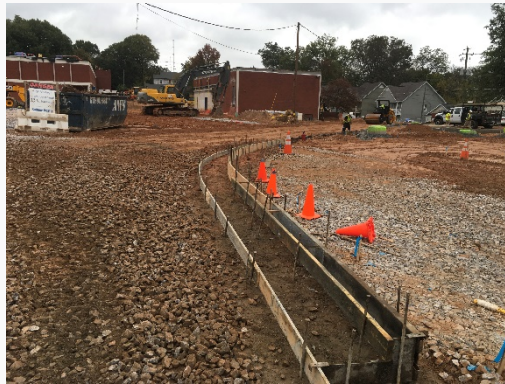
Installation of Curb and Gutter
