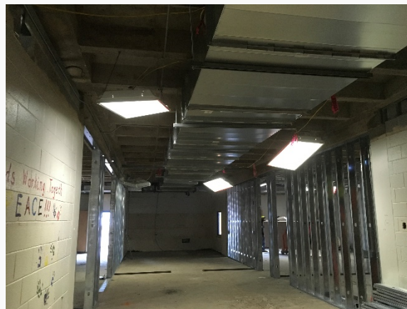
Interior MEP Rough and framing at renovation
