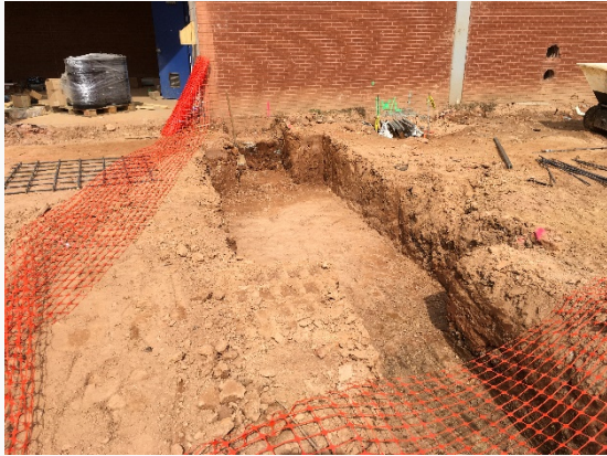
Excavation and pouring of footings
