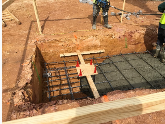
Excavation and pouring of footings
