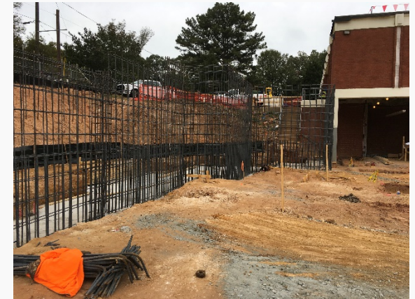
Installation of wall rebar
