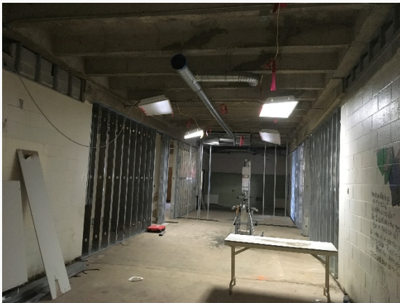
Interior MEP Rough and framing at renovation
